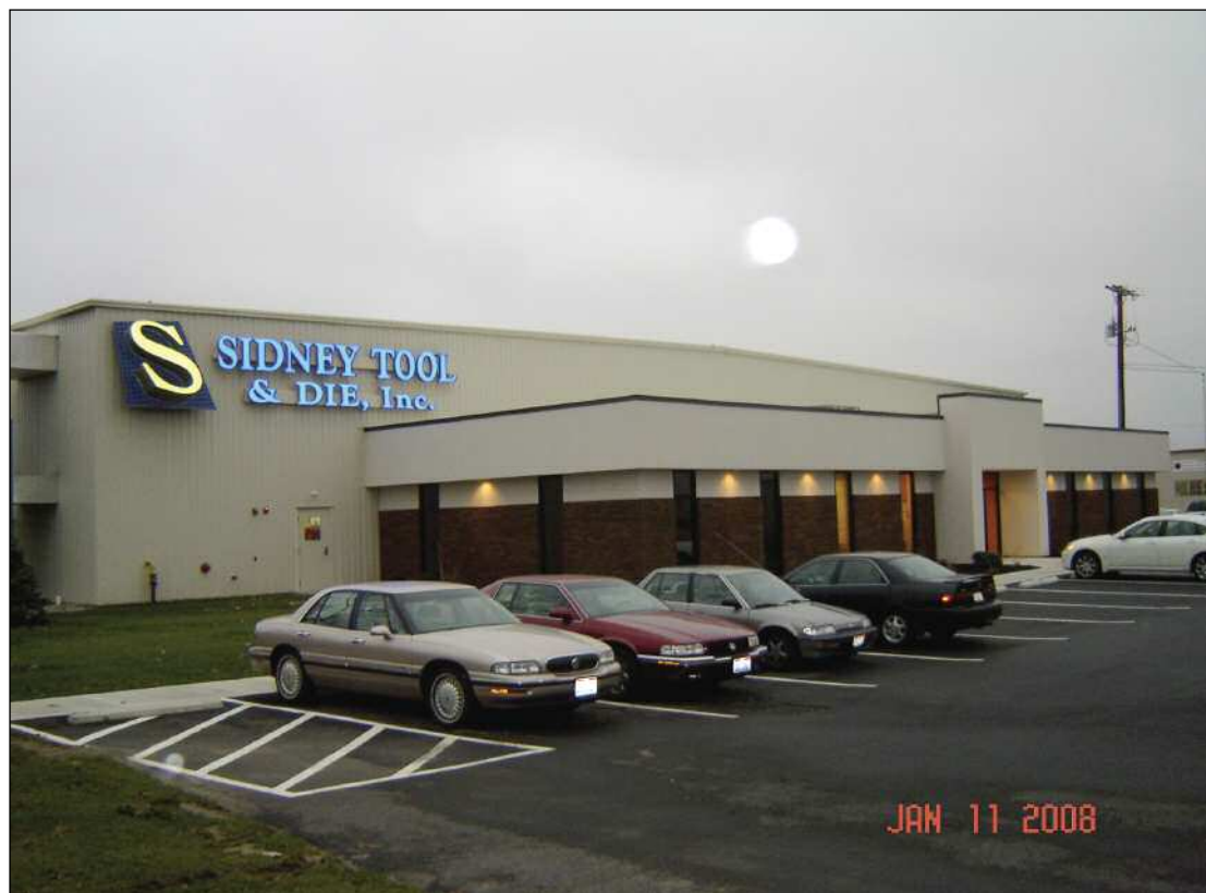
This is Sidney Tool & Die Inc.'s new 33,000 square foot new manufacturing building.
